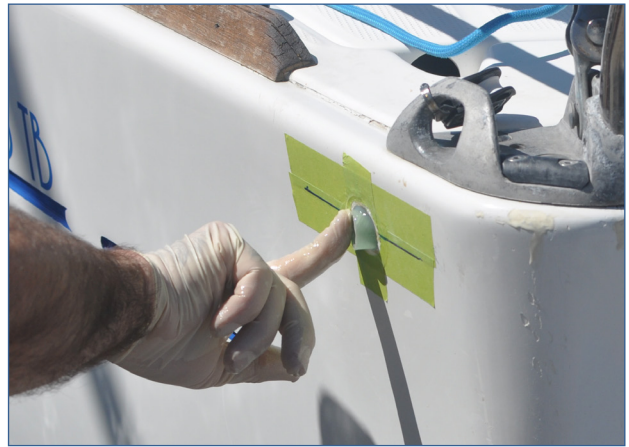
Fig 10: Make sure that there is a proper bond without voids or gaps.
