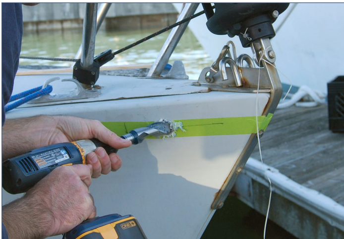
Fig 7: Drill holes using a 1" step drill.
