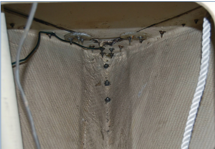
Fig. 1: Inside the hull is clear
